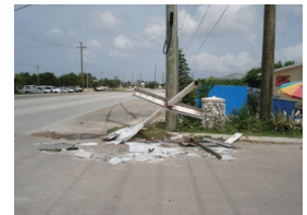
Above—original roadside sign, after demolition by a car in late June. Below—new sign.
